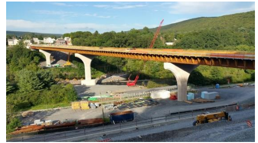
Jim Thorpe Memorial Bridge, Jim Thorpe, Pa.
